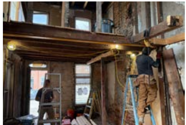
Demolition underway at 109 Schroeder Street
